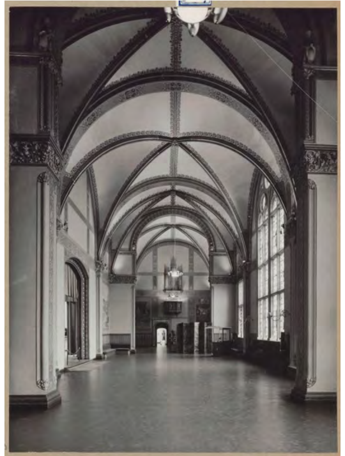
Figure 4: Great Hall, ca. 1955-57. State of the Hall after the removal of most of the decorations and wall paintings ("Overzicht centrale").
